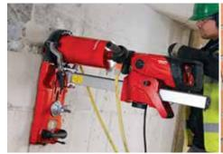
Quick and precise: wet coring in concrete using the drill stand for plumbing and heating pipe installation work.
