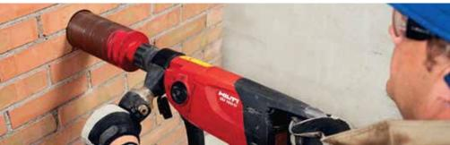
Virtually dustless dry coring in masonry with the hand-held DD 150-U.
