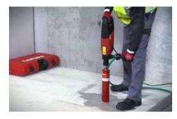
Neat and accurate: hand-guided wet coring in concrete for the installation of pipes or fixtures such as hand rails.
